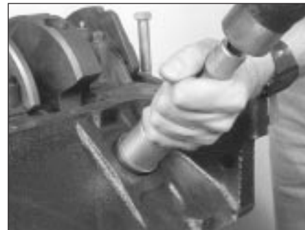
15.10 A large socket on an extension can be used to drive the new core plugs into the block
