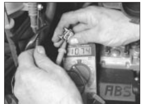
6.9 Check for battery voltage at the electrical connector to the purge valve
